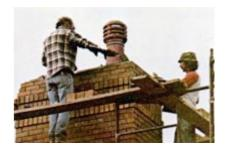
inside area of the flue liner except for the maximum 3/4 of an inch in the corners. The flue liner may extend up inside the chimney top, or the flue liner may be flush with the top surface of the chimney cap. Additional anchoring may be used to prevent damage from tornadoes, hurricanes or earthquakes. A 1/4 - 1/2 inch diameter hole may be drilled in at least two opposite sides of the chimney top and a bar used to anchor the top into the grout or the chimney walls.
